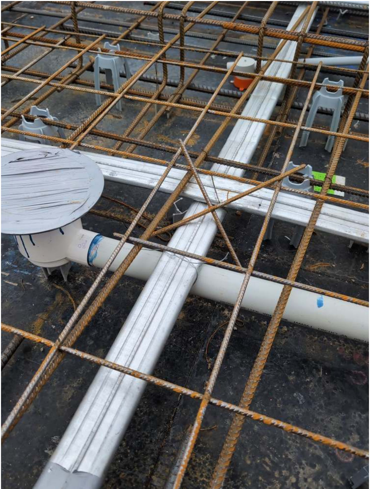
Cover between DP and PT
